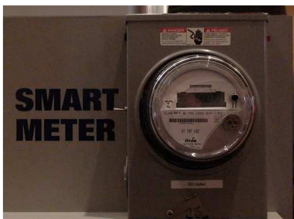
Smart Meters allow users to monitor their energy usage in real time, to donate renewable energy back to the grid, boosting the nation's supply, and to manage the power sent to appliances. Photo by Tom Raftery. (License: Creative Commons Attribution-Non commercial-Share Alike 2.0 Generic)
